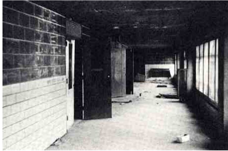
Figure 6: Pruitt-Igoe Shared Galleries, conceived as "indoor streets"
